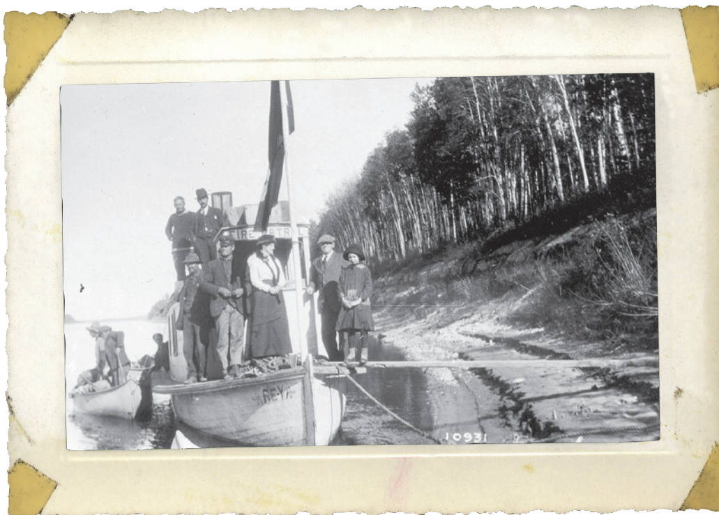
Fire patrol boat, the SS Rey, on the Athabasca River, near Athabasca, Alberta, 1916. This boat was based at Athabasca Landing and patrolled between Grand Rapids and Mirror Landing. It was 42 feet in length with a ten inch draught and a powerful engine to force the boat upstream against the fastest current. The skipper was the fire ranger and had a crew of an engineer, a fireman-stoker and whatever help was occasionally required. Patrol boats were on the alert for lightning strikes and campfires left by travellers who used the rivers as highways to the north.
